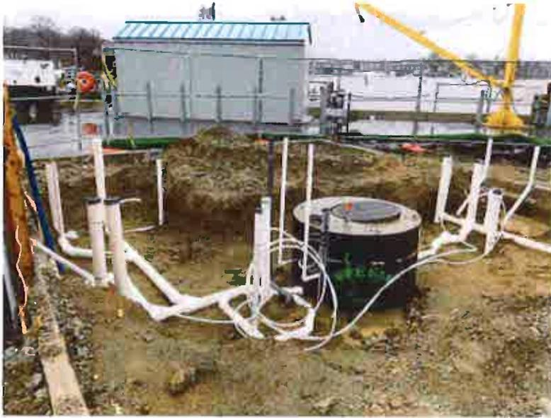
*Photo 1: Wet well and underground piping arrangement, looking north.*
