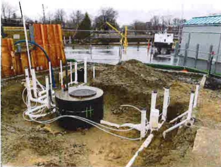
*Photo 2: Wet well and underground piping arrangement, looking west.*
